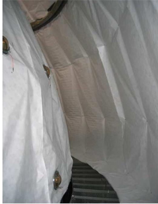
Fig. 5. The inner surface of the Water Tank covered with layer of Tyvek. The Tyvek sheets improve light collection in the Outer Detector by reflecting the photons back into the water.
