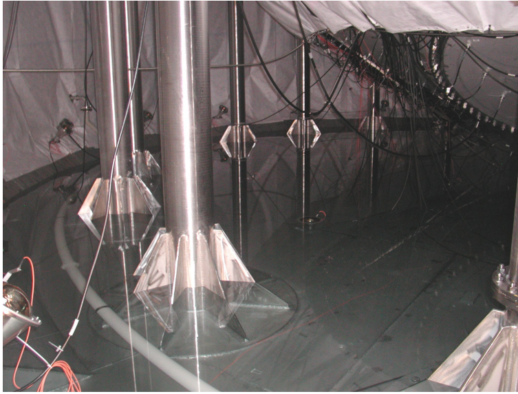
Figure 2.3: Picture showing the outer detector: The inner walls of the dome and the outer side of the Stainless Steel Sphere. It also shows the up and inward pointing PMTs and some of the legs carrying the SSS. The picture was taken during filling process [BorWP].
